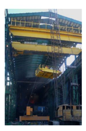
There will be no any flame cutting and welding at site during our World-leading cranes installation. Reliability lifting belts will be serviced for any lifting, cranes surface will be really protected by soft belts. Our bolts connection design has renovated site job, flame cutting and welding will be replaced by toque spanner in our teams.
